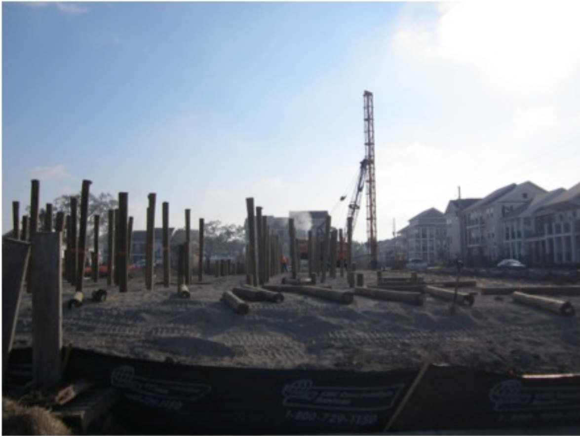
Construction begins at the Columbia Parc IIB site.
